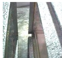
Blower Section (left) and bottom of coil (right) with \frac{3}{4} " slot.
