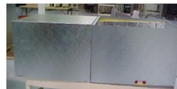
Front of blower (left) connected to a HD coil (right).
