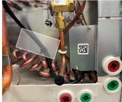
3. Install the provided split grommet in the coil panel, reinstall the panel, and route the sensor cable through the grommet.
