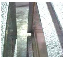
Blower Section (left) and bottom of coil (right) with 3/4" slot.
